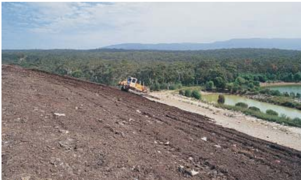
Above: Greenwaste from the City's transfer stations and on-call service is mulched and composted under contract by Soilco at their purpose-built processing facility in Nowra. Below: A percentage of the composted material is utilised at the West Nowra Landfill as part of the revegetation process for filled and capped cells.
